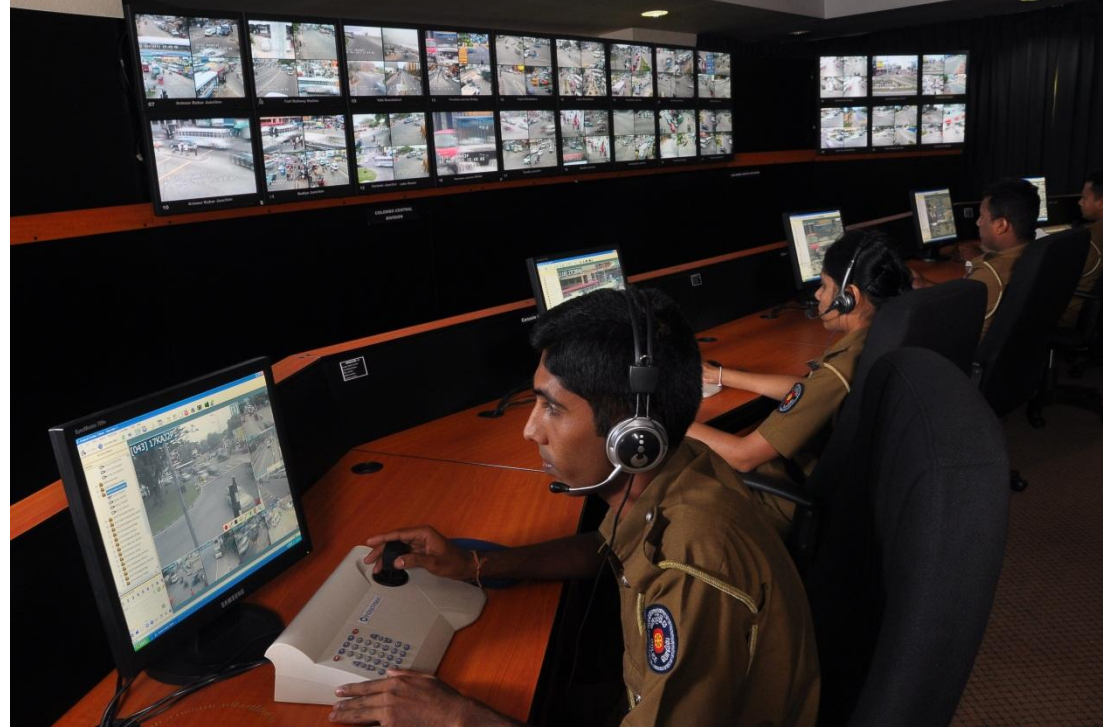
Central Control Room
